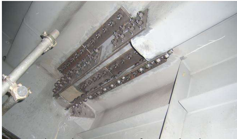
Partial replacement of trough rib For DS, FR cracks
