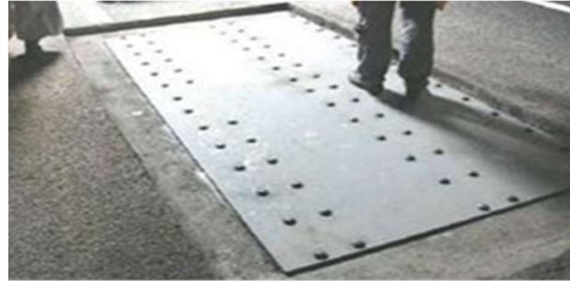
Patching steel plate
