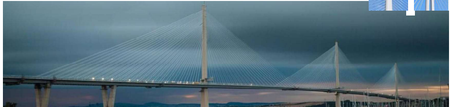
Four span cable-stayed bridge, 650m Queensferry Crossing Bridge 2017
